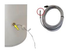
Replace protective cap and seal hole with sealant. Clamp cable to storage tank to prevent movement of sensor.
