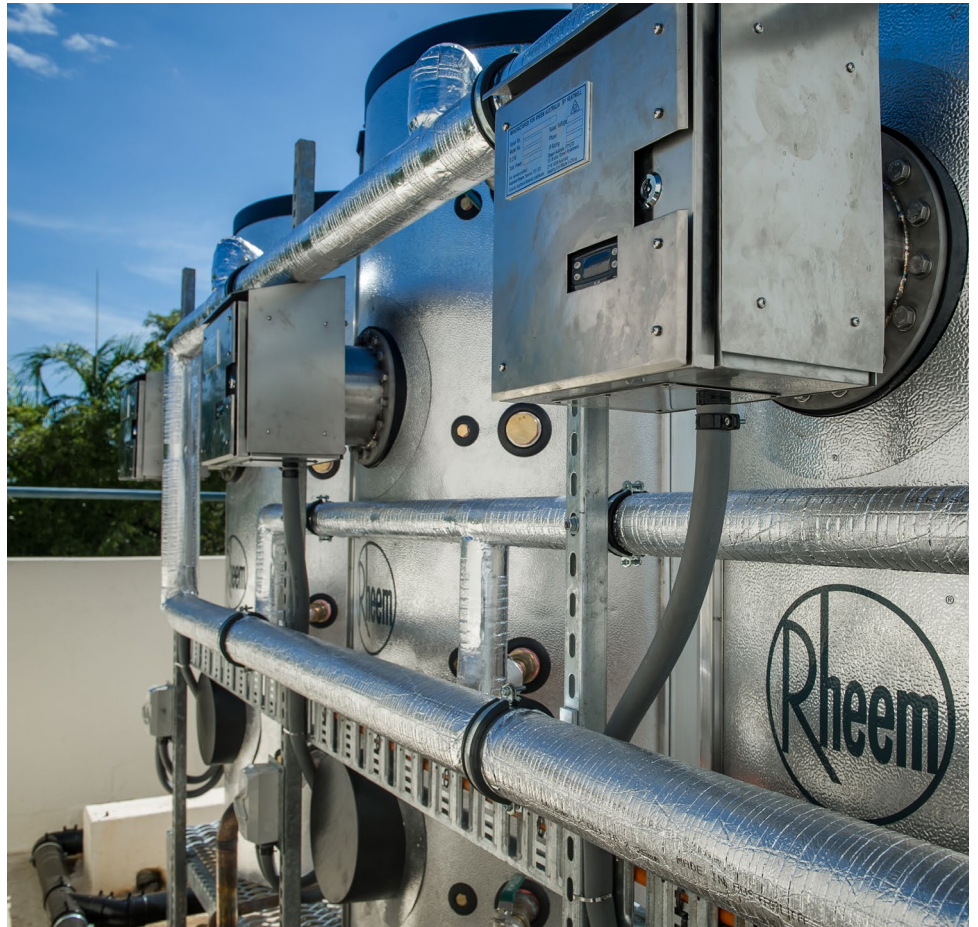
Rheem HS Series solar with electric boosting in the top of solar tanks. Katherine Hospital NT.
