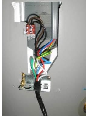
Step 3 withdraw the power cable
