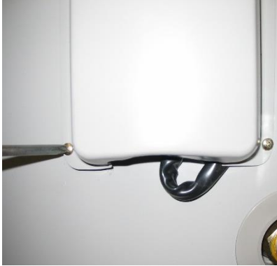
Step 2 remove screws from lower front cover
