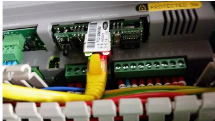
Status GREEN- card communication OK Ethernet RED- No connection between card and network
